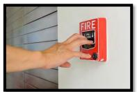
General Description: Fire alarm systems consist of manual and programmable pull stations, visual/audible alarm devices, addressable smoke detector/sound bases and smoke/heat detectors in individual sleeping rooms, corridors, common area and mechanical spaces.
